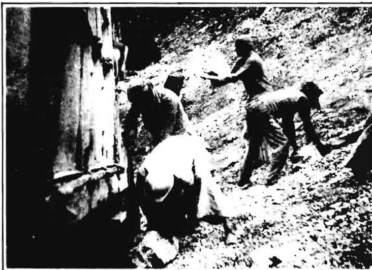
Loading Limestone: Clandestine operations
